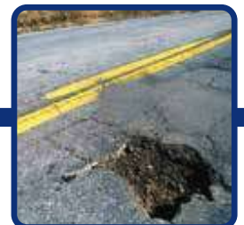
POTHoles/DAMAGED PAVEMENT
